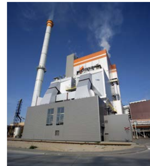
Our new recovery boiler at our Świecie operation (Poland)
