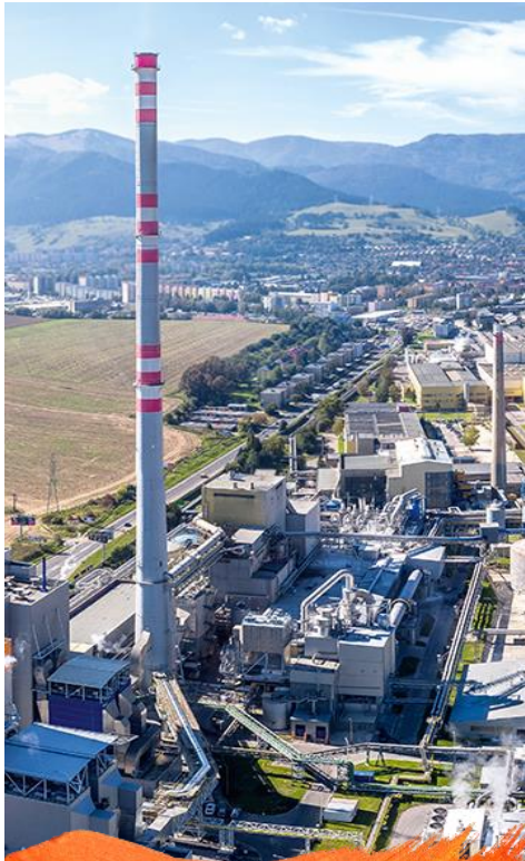
Ramping up new containerboard machine at Ružomberok (300ktpa)
