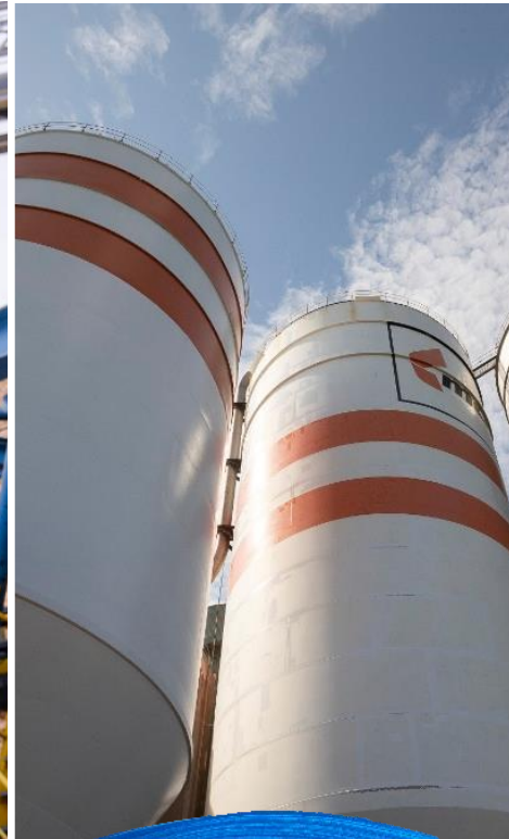
Modernisation of Richards Bay
