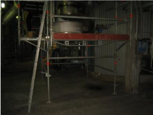
Safe access ladder (4:1)
