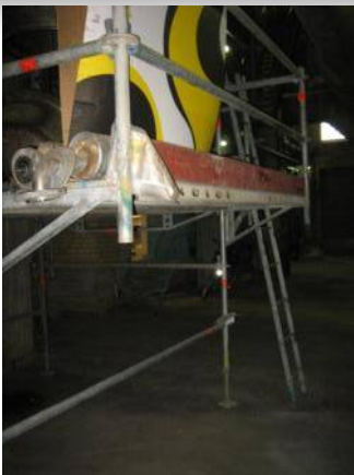
Toe boards & railings
