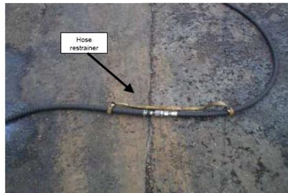
Figure 12: Restraining a Hose Joint
